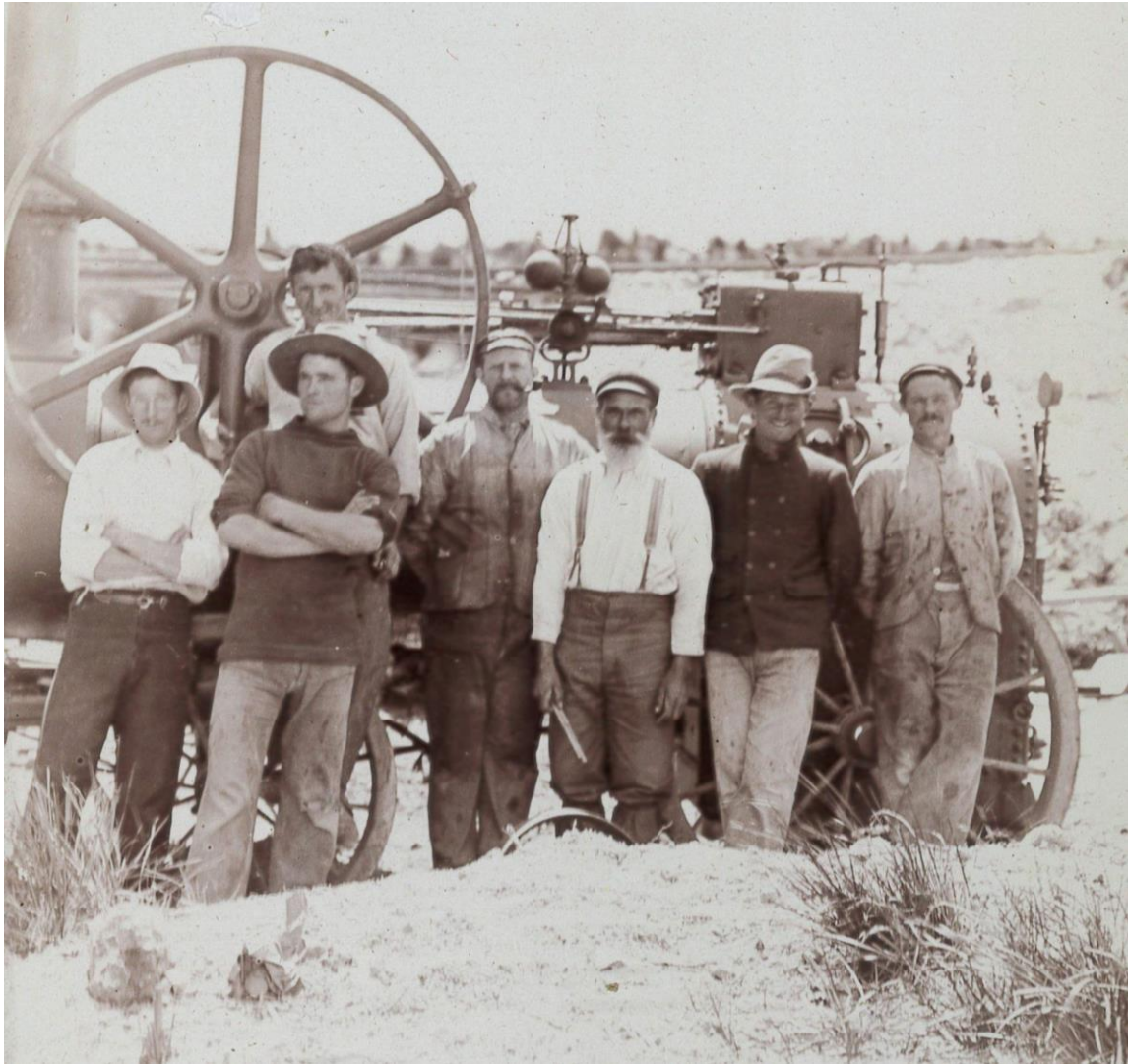
China stone and clay mine hands assembled beside the boiler showing its fuel regulator or centrifugal governor 'balls', flue and fly wheel. Joseph (Joe) Seymour (in braces) became the father-in-law of Frank Abell who worked as a potter at Penneshaw's brickworks (J.C. Radcliffe Collection).
