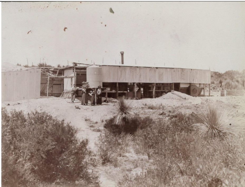
The china stone and clay mine. Water from the windmill was piped across into the machinery shed. Is it a basalt roller leaning against the shed, and an experimental brick wall, top right? The mine, at the lowest level of the basin-like grounds, gave gravitational access to trucks running from the diggings (J.C. Radcliffe Collection)
