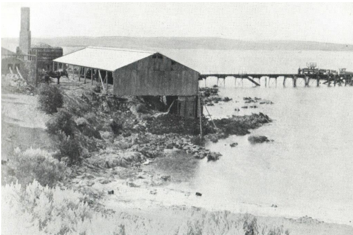
Penneshaw brickworks and jetty. View northwards. The mainland lies on the horizon. Probably 1908 (State Library of South Australia, B 50426). 'The works ... consist of a manager's office, engine house, two drying sheds (one 60 feet by 27 feet and the other 100 feet by 30 feet) a circular kiln which will hold about 23,000 bricks and a new kiln in course of erection which, when completed, will hold 35,000 bricks.' (Unohoo, 'Kangaroo Island China Stone and Clay Company', Kangaroo Island Courier , 3 October, 1908, p6a).
