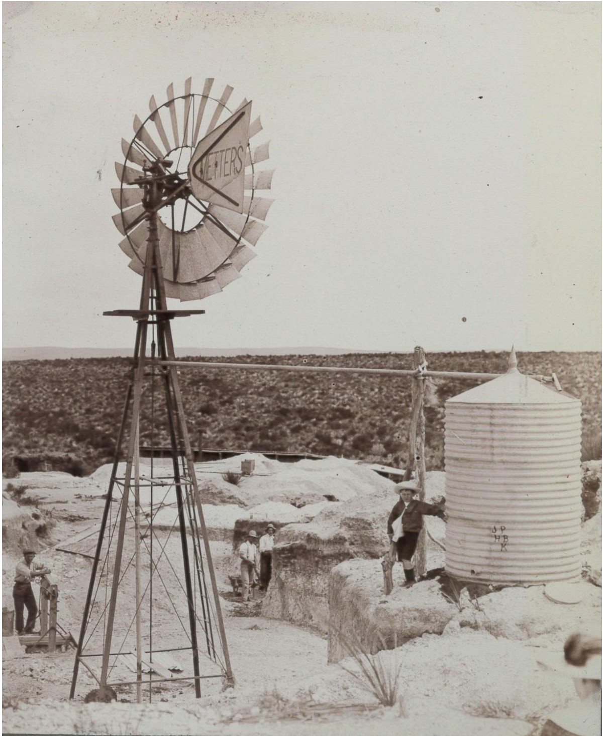
Open-cut mine and water pumping station, looking south. Fred Metters (1858-1937) began manufacturing water-pumping windmills at Adelaide with his 'Windmotor' in 1896. A shed runs behind on the perimeter. A few rail lines are laid. The woman in a hat in the lower right corner was no doubt a companion of the photographer. The tank is initialled JP/HB/K which John Radcliffe in a personal communication thinks with reason stands for John Provis, Hog Bay, Kangaroo Island (J.C. Radcliffe Collection)
