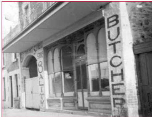
The 'Gilbert Street Meat Store, Quality Butcher' later became 'Cimarosti and Sons Quality Meats'. The building's front was changed by 1971, leaving little indication of the original nature of the archway for the butcher's horse and cart. (Courtesy of Julie and Steve Cimarosti)
