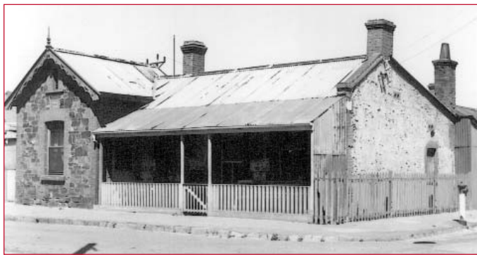
No. 1 Mary Street, formerly on the corner of Alfred Street. Murray Cartwright, who was born in the cottage in 1943, then the only one in Mary Street, recently returned to the South West to establish an exhibition gallery in Sturt Street. (Courtesy of Murray Cartwright)
